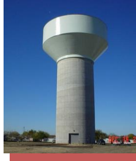
Water System Development
